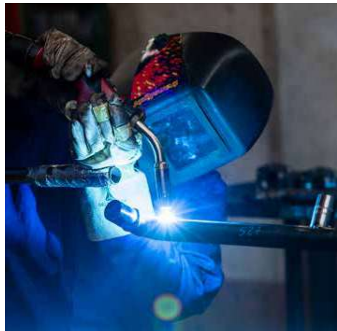
Carbon and stainless-steel welding by Hydroalp
